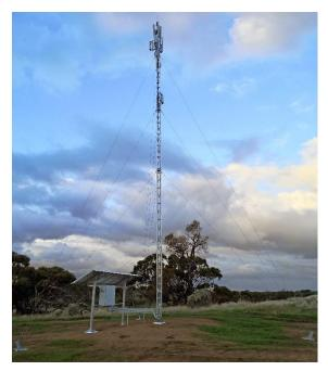
The ground mounted AL220 tower series are recommended to be used in conjunction with Surefoot Footings for a simple, concrete-less installation. Concrete cages, skids, and other options are available on request.
