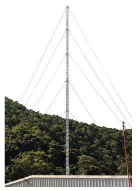
Your safety is most important - the tower base comprises of a 50 tonne rated, fully machined billet aluminium universal-joint. This universal-joint design allows axis locking to permit safe and easy raising, as well as the components machined from solid structural grade aluminium providing absolute peace of mind of tower integrity.
